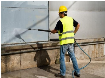
Cleaning Tunnel Walls
